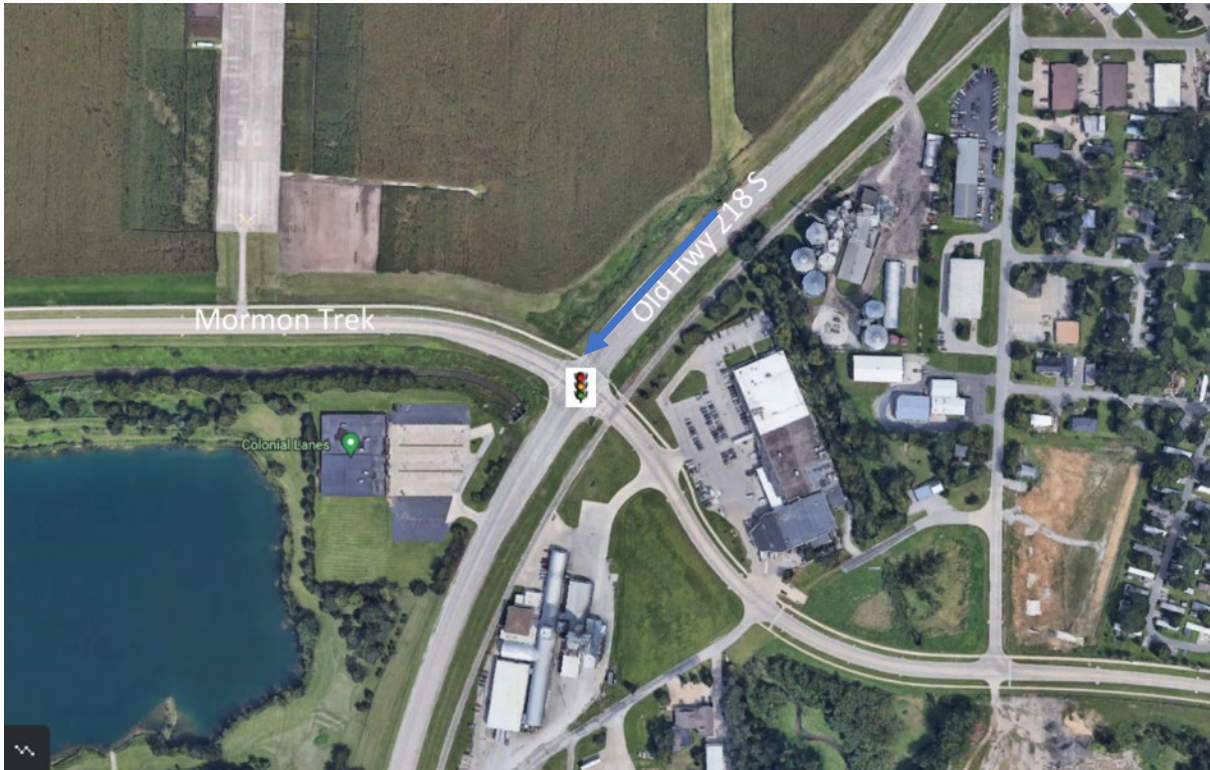
Figure 18. Traffic signal at Old Hwy 218 S and Mormon Trek Blvd
